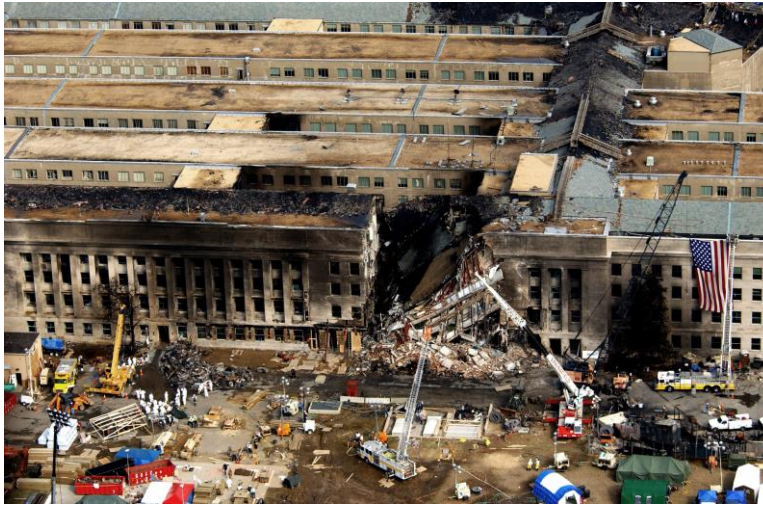
Caption #2: The Pentagon partly-collapsed due to impact and fire damage after 9/11 attack
